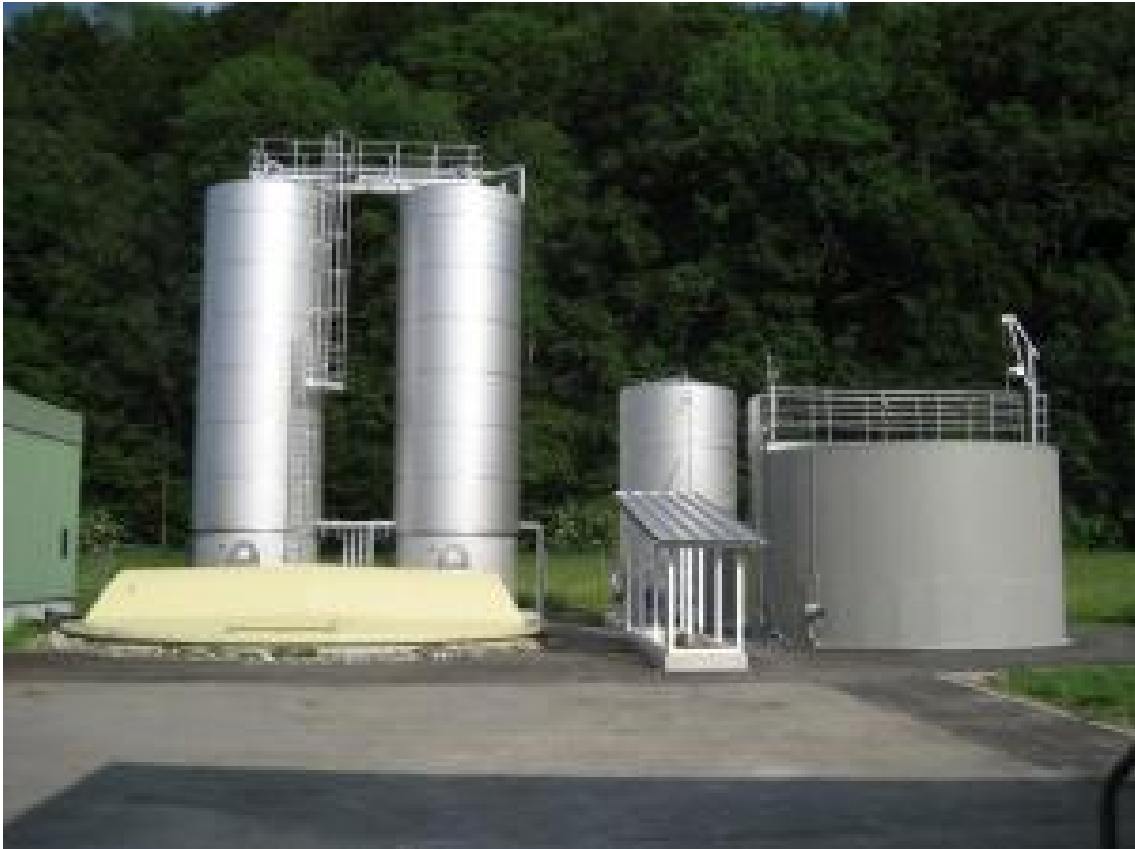
Sewage plant in Schwerzen. This 10,000-strong municipality has already opted for high-rate digestion. (Credit: Copyright Fraunhofer IGB)
